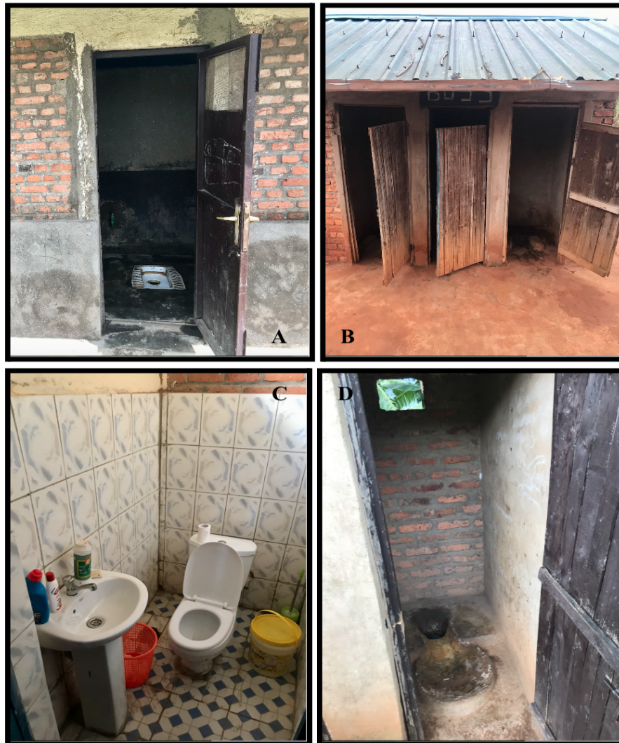
Figure 4. Sanitation facilities in lower secondary schools in Rwanda. A. Pit latrine with locking doors at a government aided school. B. Pit latrine with a non-locking, non-closing door, and no ventilation window at a public school. C. Flush toilet, sink with running water, soap, waste receptacle, and toilet paper in MHM room at a government aided school. D. Pit latrine with a non-locking door at a private school. Photo: Kirsten Dodroe, with permission.
